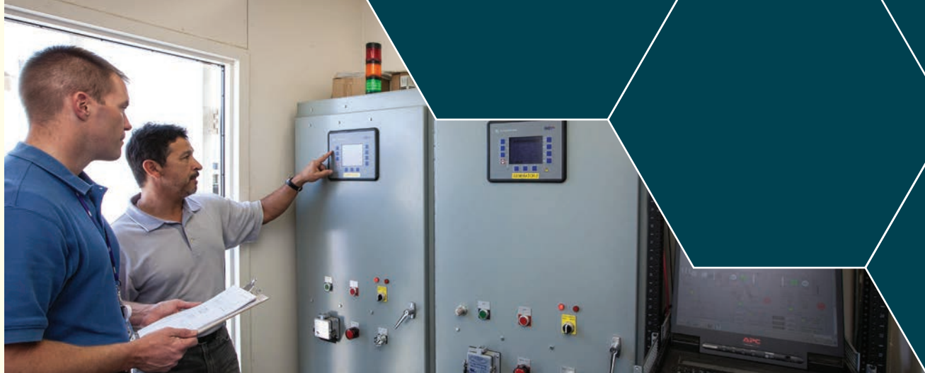
Neal Bartek (left), San Diego Gas & Electric (SDG&E) smart grid projects manager, and Gil Montes (right), who serves as a project manager with the company, inspect the controls unit for on-site generation at the Borrego Springs microgrid operated by SDG&E.
