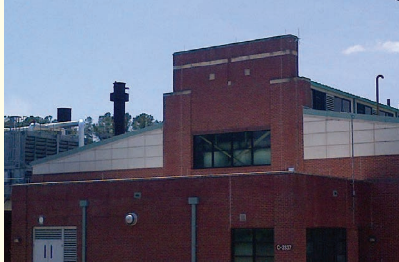
Photo of the 82nd Airborne Cogen Plant at Fort Bragg—one of the generation assets that will be tied into the microgrid.
